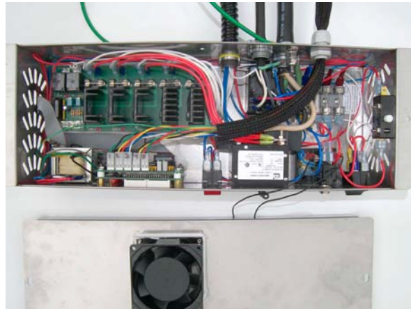
3 Gp, June 2006: Tyco pump relay, SPF relays on zones 4 & 5 for 2 gp machines
